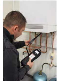
Ambient CO checking
